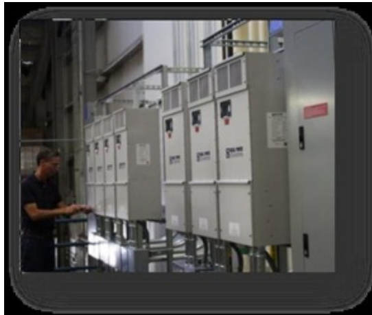
Figure 6: Seven of our 30kW PV Inverter in use at the University of Texas- Austin
