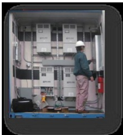
Figure 7: Our 30kW battery converter used for containerized grid energy storage undergoing testing at the Bonneville Power Authority, Washington
