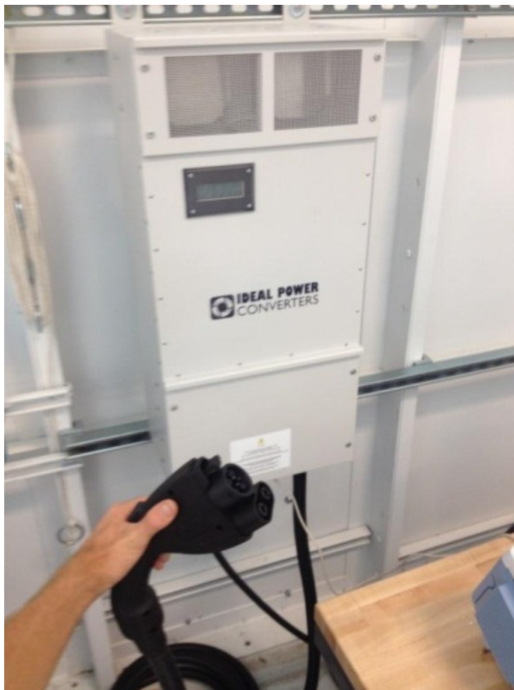
Figure 8: Our 30kW battery converter used for bi-directional DC charging at the National Renewable Energy Laboratory, Colorado
